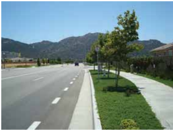
View of vault located in grass, looking West.
