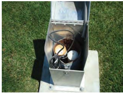
View of wells inside vault.
