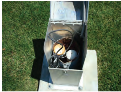
View of wells inside vault.
